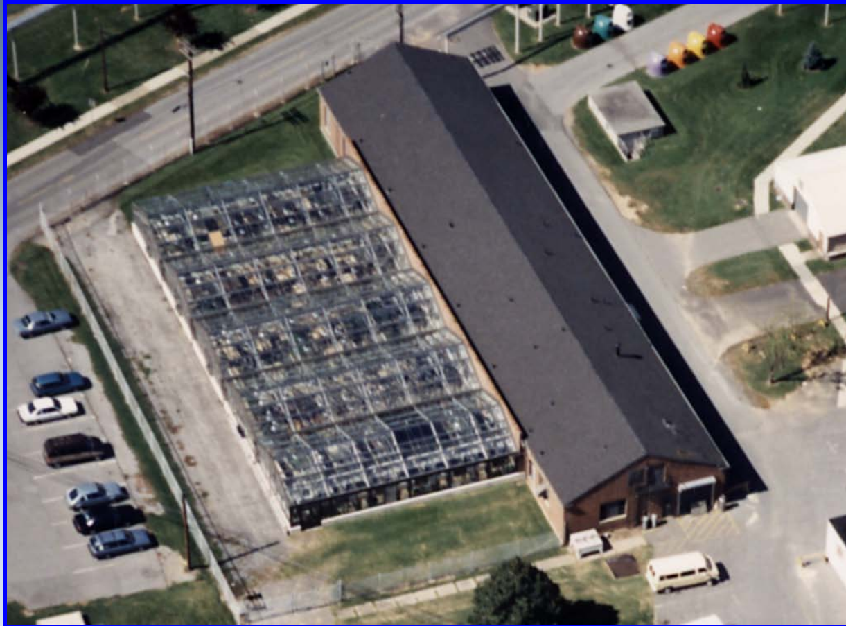
The Containment Greenhouse Facility
